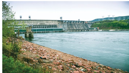
Hydro power plant
